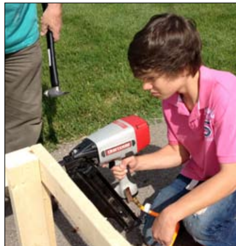
Austin Binder, 15, volunteers his time building camera platforms for the North Campus video equipment installation.
